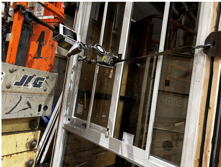
Photo No. 22 Forced Entry Resistance Testing
